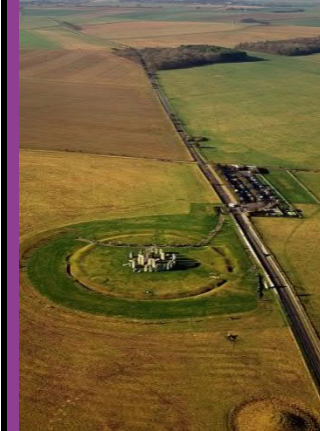
A303 Stonehenge Road Tunnel, UK
